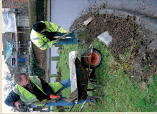
Repairing lorry damage
